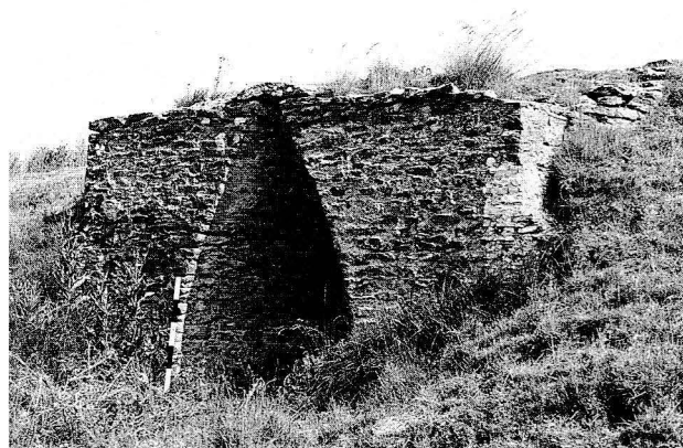
Plate 2. New Lane, Swyre. A small pointed arch Type C limekiln. July 1993.
