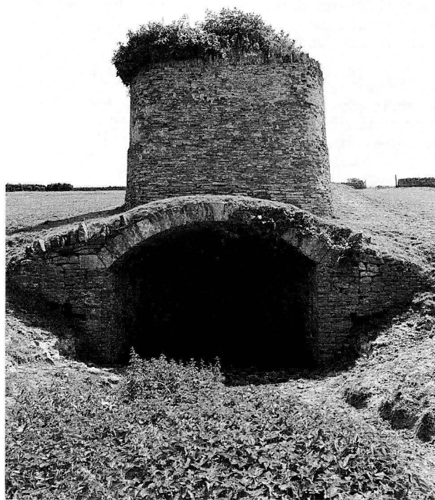
Plate 4. Whitmore Coppice limekiln from the north, showing the unusual tunnel approach to the draw arch area. June 1993.
