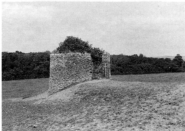
Plate 3. Whitmore Coppice limekiln at Langton Herring from the south, showing the retaining wall (restored) around the kiln head and pot. June 1993.
